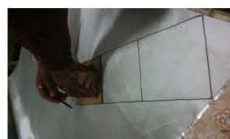
Fig. 1. Marking the fiberglass sheets of 45° orientation
