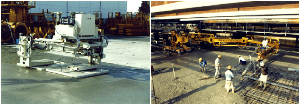
Figure 2: (From left to right, respectively) Concrete Surface Treatment Robot and Concrete Horizontal Distributor [3]
